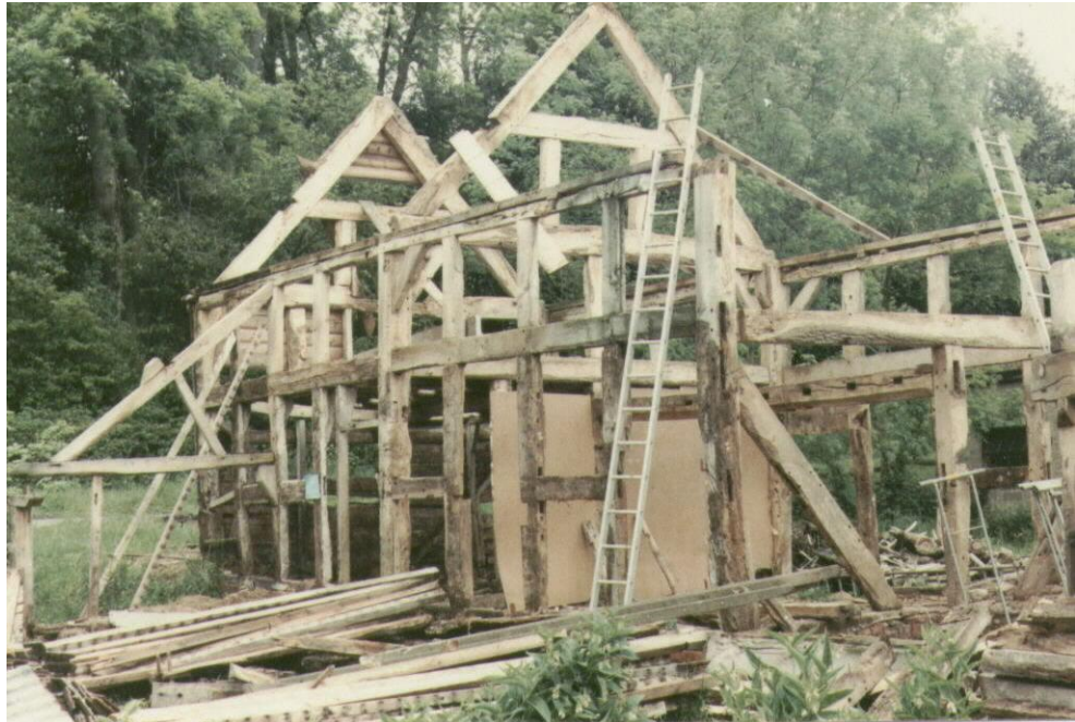
Dismantling the barn at Oldfield Farm
