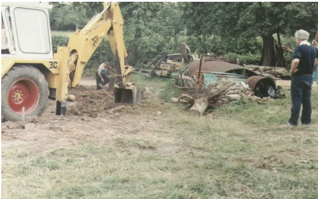
Preparing the site in the orchard of Tudor House
